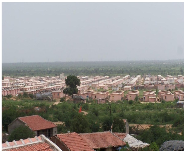
A relocated village in Bhuj, Gujarat
